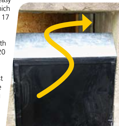
Photo 17 : Lateral chicane consists of a partition which guides bats to a room on the right side (roost Am11).
