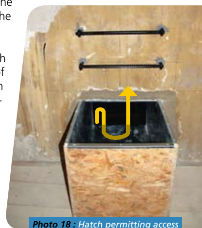
Photo 18 : Hatch permitting access for bats to the attic (roost G04).
