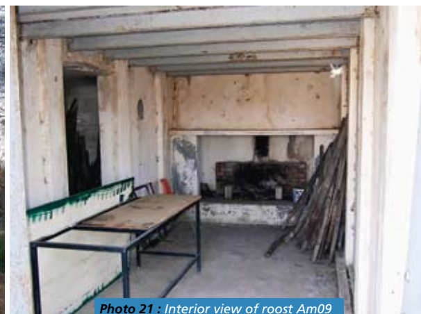
Photo 21 : Interior view of roost Am09 before development.
