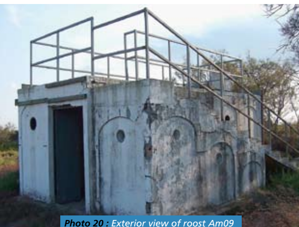
Photo 20 : Exterior view of roost Am09 before development.
